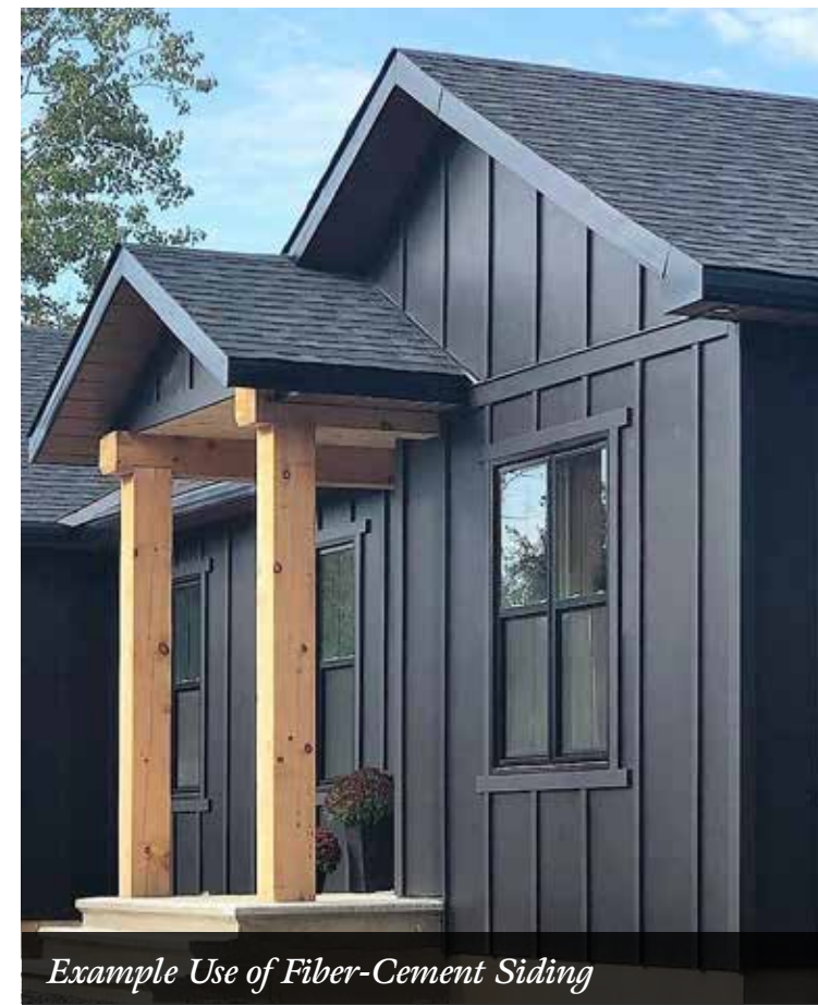
Example Use of Fiber-Cement Siding
