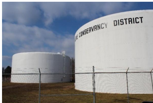
Above ground water storage tanks are used to ensure water is available during times of emergency.
