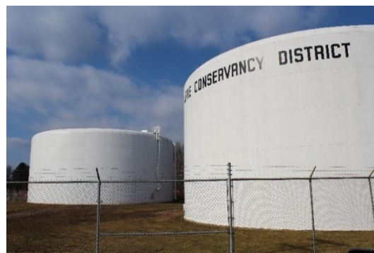
Above ground water storage tanks are used to ensure water is available during times of emergency.
